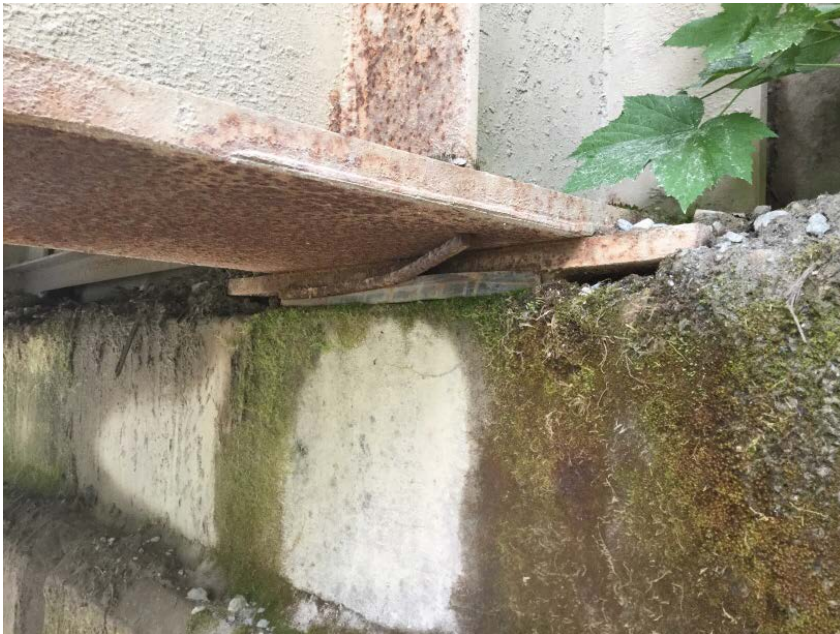
Right upstream bearing pad keeper condition
