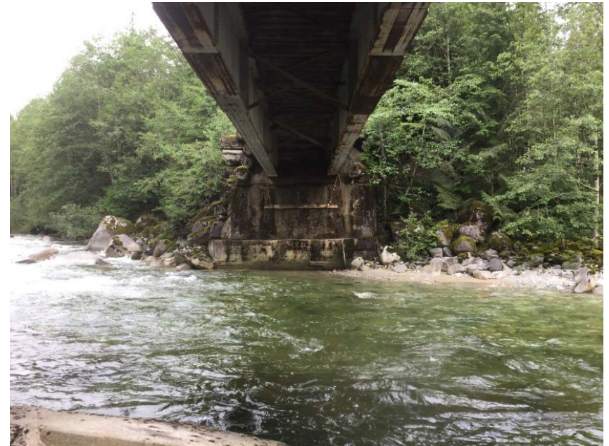
Left Bank Abutment when facing downstream
