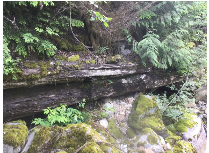
Log wingwall at left downstream location
