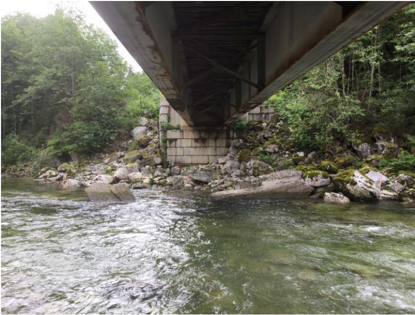
Right Bank Abutment when facing downstream
