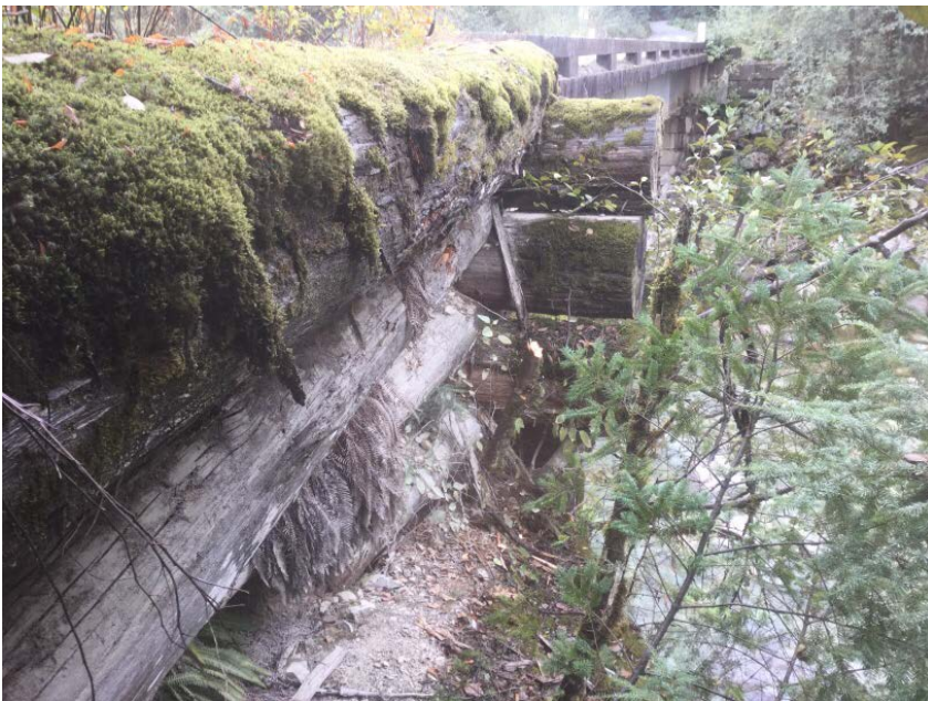
Log wingwall upstream left bank
